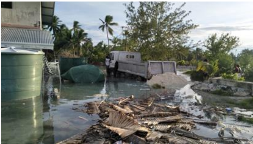
Truck bogged while repairing Kiribati Health Retreat's broken seawalls following Cyclone Mona in January this year. Photo courtesy Pelenise Alofa
