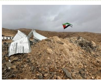
The destroyed school of Isfey al Fauqa 2 days later.
