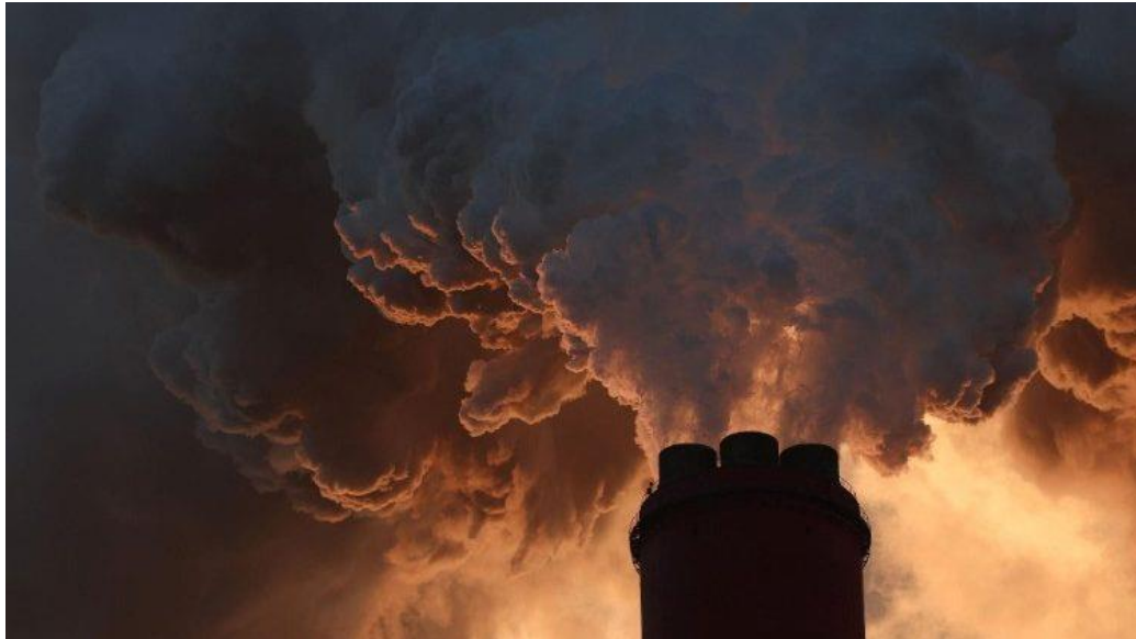
Smoke billows from Europe's largest coal-fired power plant
